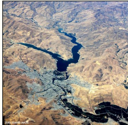
Mahabad dam, Iran
