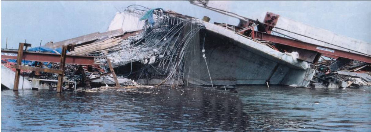
Fig. 10. Collapse of a bridge due to lacking control of the specific ground properties during pile execution (no comparison of design assumptions and locally found soil).
